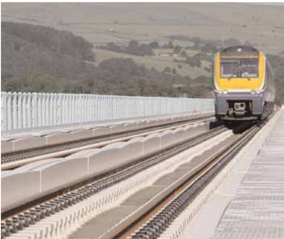
PANDROL VIPA-SP baseplates installed on a steel deck bridge
