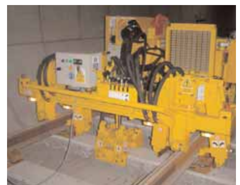
Mechanised installation of pre-assembled PANDROL VIPA-SP baseplates
