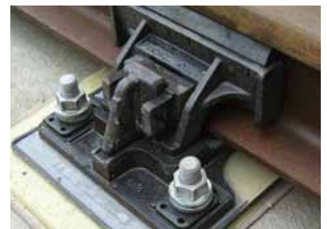
Baseplate VANGUARD assembly installed on concrete slab
