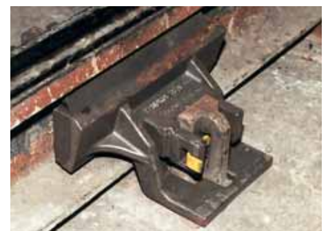
Cast-In PANDROL VANGUARD assembly installed on concrete slab track
