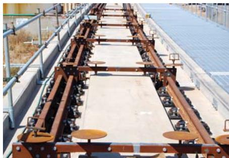
Iron horses used to level and align track Prior to grouting of VIPA-SP assemblies
