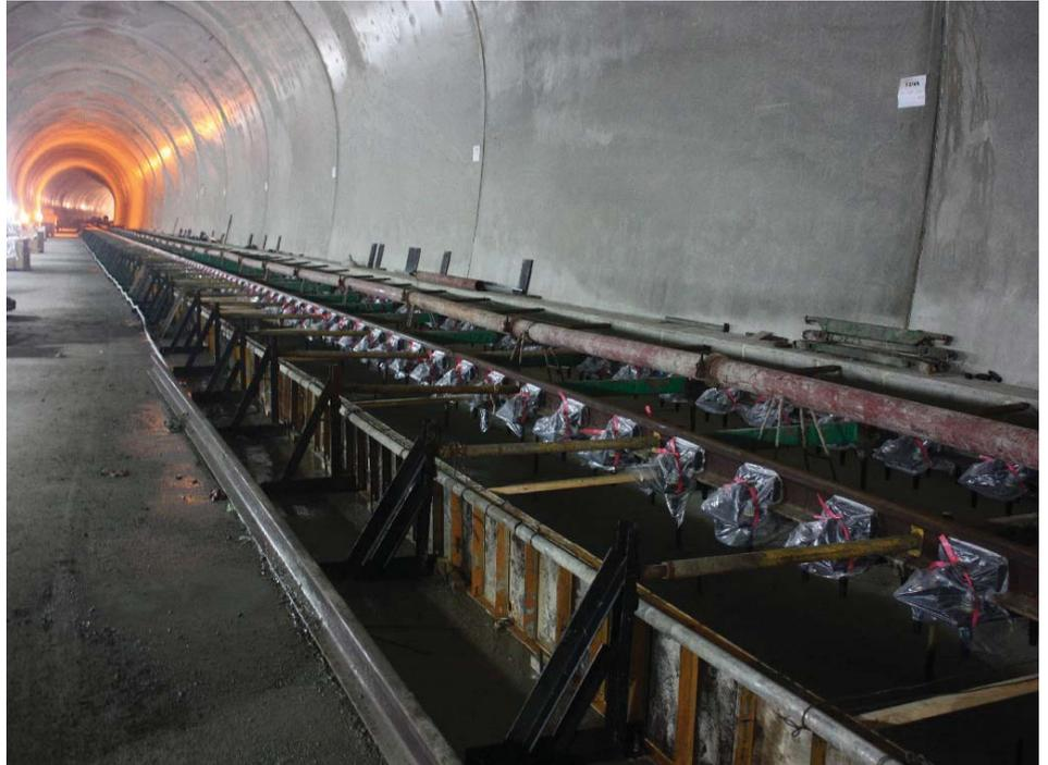
Track with VANGUARD fastenings prior to concrete slab pour
