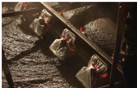
VANGUARD assemblies are protected during the concrete pour to prevent ingress of concrete into the fastening
