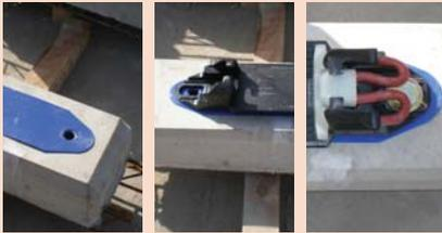
2. The pre-assembled baseplate was bolted to the twin-block sleeper, with a conforming pad beneath the baseplate.
