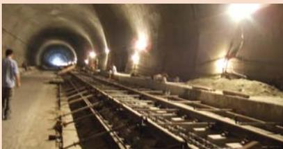
3. The twin-block sleepers complete with fastenings were laid onto the tunnel base slab and top slab base reinforcement.
