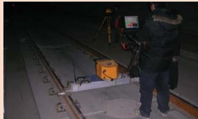
5. In between materials trains, a full line and level survey of the rails was undertaken using very accurate rail mounted laser based equipment.
