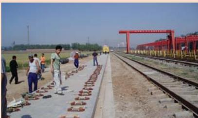
2. The baseplates were fitted to the slabs in the 'neutral' position.
