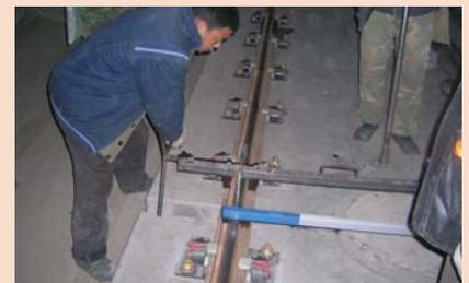
11. Lateral adjustment then took place. After loosening the baseplate bolts on the datum rail, engineers could crowbar the rail to the amount required and make the adjustment using the slots in the baseplate and the serrated washer. The datum rail baseplates were then tightened and the gauge set on the other rail in the same manner.
