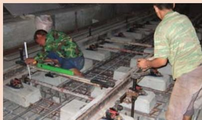
5. Spindle jacks were fitted to the rails and the rails were lifted, lined and levelled. The rails were fitted with Gauge Bars to prevent the rail gauge decreasing due to bending of the twin-block sleepers.
