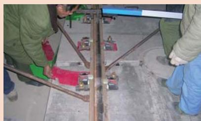
7. An adjustment team followed behind. A series of colour coded LDPE, HDPE and steel shims were provided, which allowed the track height to be very accurately set. Baseplate bolts could be loosened, the rail lifted with crowbars, and the correct shims slid into place.
