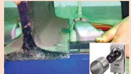
8. In case of any suspensions of rail base in some rail seat areas it's also important to check the gap between the datum surface of baseplate and the bottom of the rail base, using a simple 'gap gauge' to measure the gaps. An alternative way can be a measurement using a laser measuring device.
