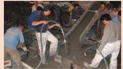
6. Once the track had been precisely adjusted, concrete was poured to form the final track.
