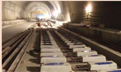
4. The rails were threaded into the rail seats, and the clips applied.
